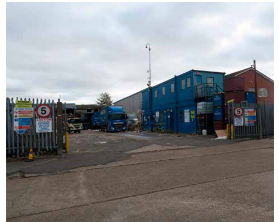
05 Existing Site Entrance
